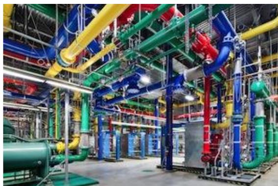
**Big data means big servers and big cooling requirements.** Google's colorful pipes carry water in and out of one of Google's data centers. The blue pipes supply cold water and the red pipes return the warm water back to be cooled.
